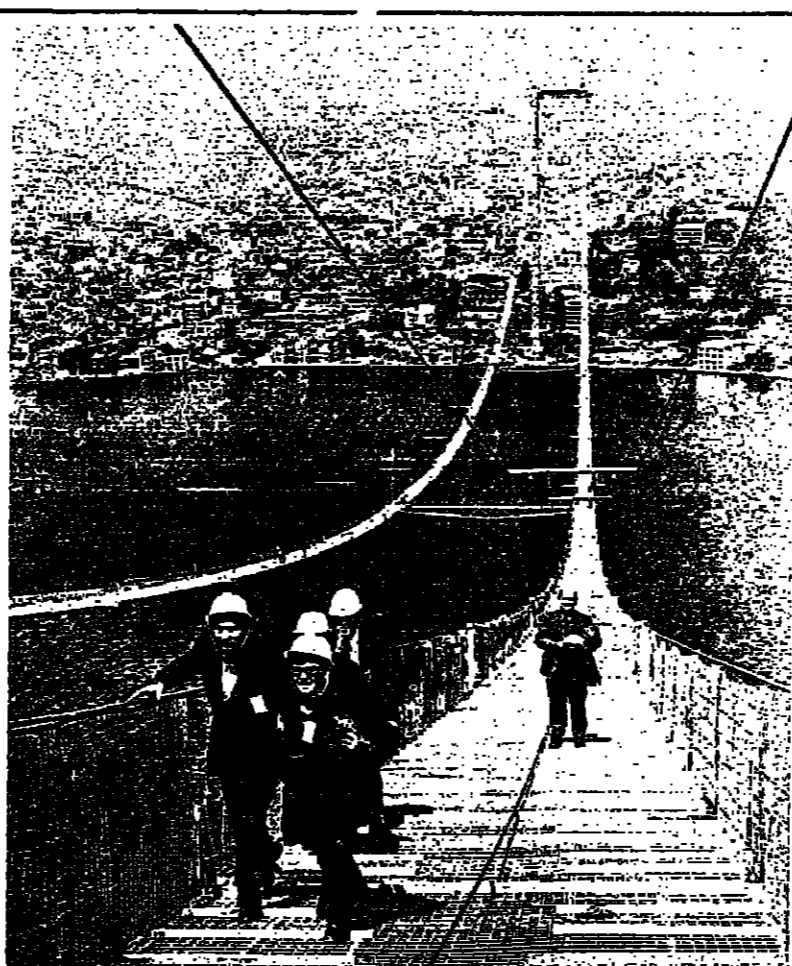
Turkey's $75.9m. first intercontinental suspension bridge is well on its way, and is due to be completed in 1975. The bridge will connect Asia and Europe over the Bosphorus, a distance of 1.6 kms. It is being built by Anglo-German and Japanese firms. (Keynotes, Israel Sun)
